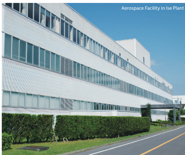
Aerospace Facility in Ise Plant
